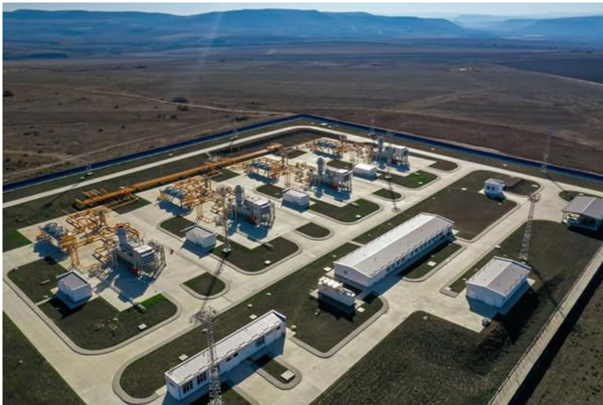
Compressor Station Nova Provadia
